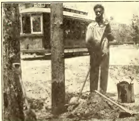
Superficial Treatment Applied to Installed Pole
