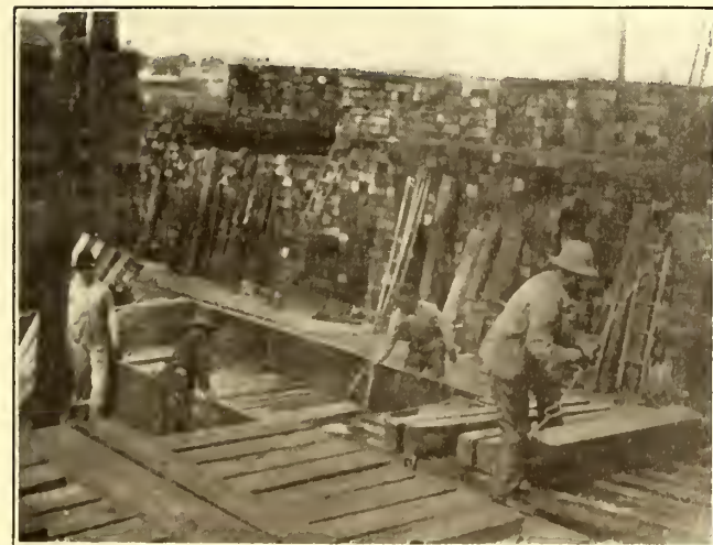
Tie-Treating Plant in Denver
