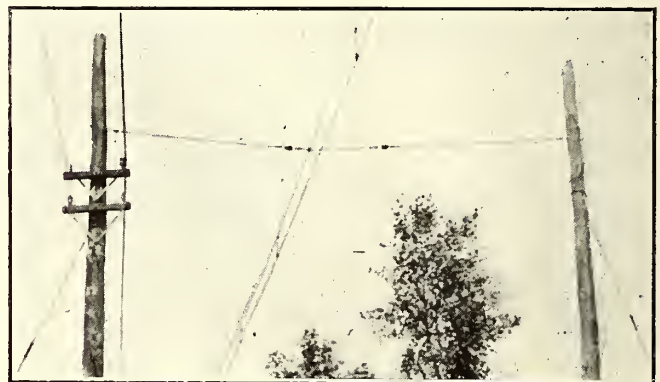
Elmer P. Morris Company's Span Work
