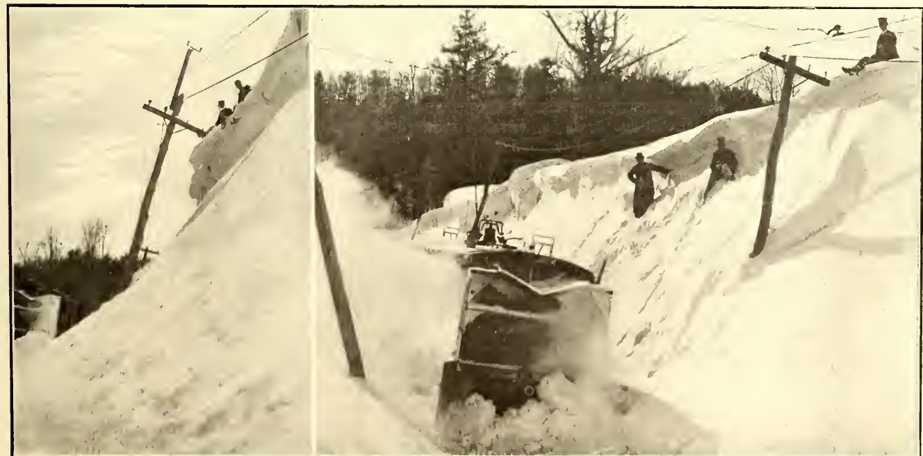
Views Showing Snow and Rotary Plow on Otsego & Herkimer Railroad Four Days Before Thaw Commenced—The Snow Bank Illustrated in the Left-Hand View Was 47 Ft. High.
