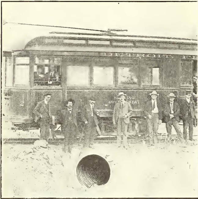
Corrugated Iron Culvert Pipe, 36 in. in Diameter, with Shallow Cover Supporting Interurban Car Without Deflection
