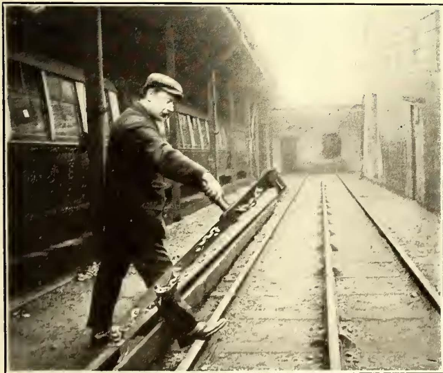
London Underground Railways—Motorman's Short-Circuiting Beam
