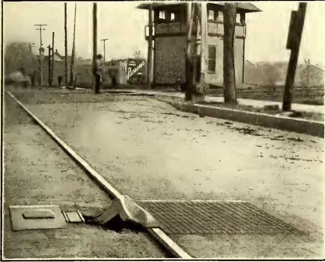
Derail in Closed Position on the Rail
