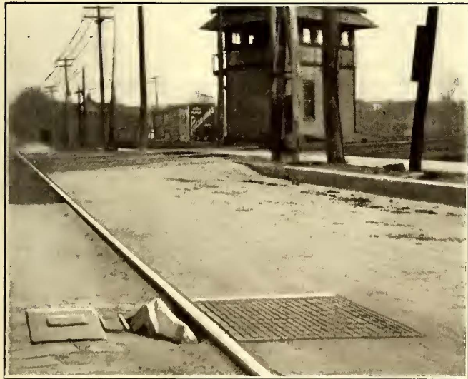
Derail Operated by Pipe Line from Tower
