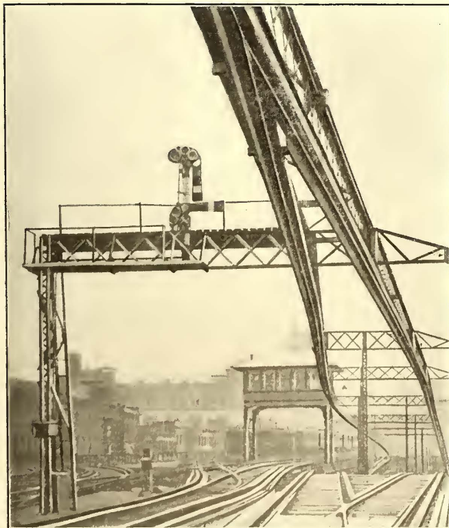
Brooklyn Line Department—Iron-Bar Construction on Brooklyn Bridge Surface Car Incline
