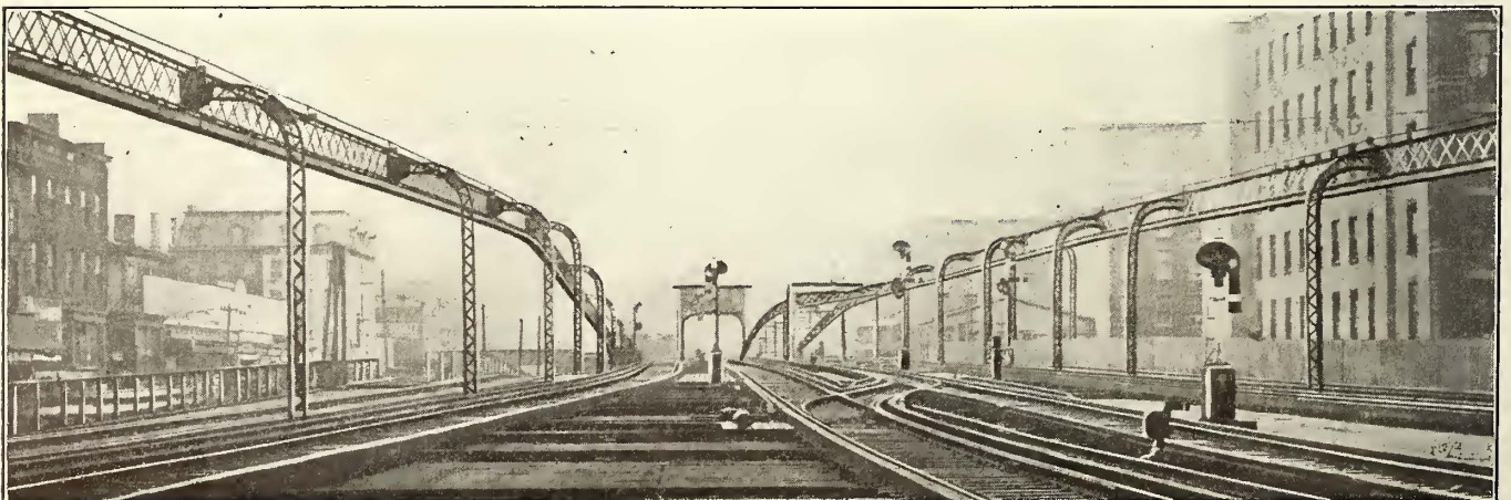
Brooklyn Line Department—Iron-Bar Construction from Davit Trusses, Looking Toward Brooklyn Borough
