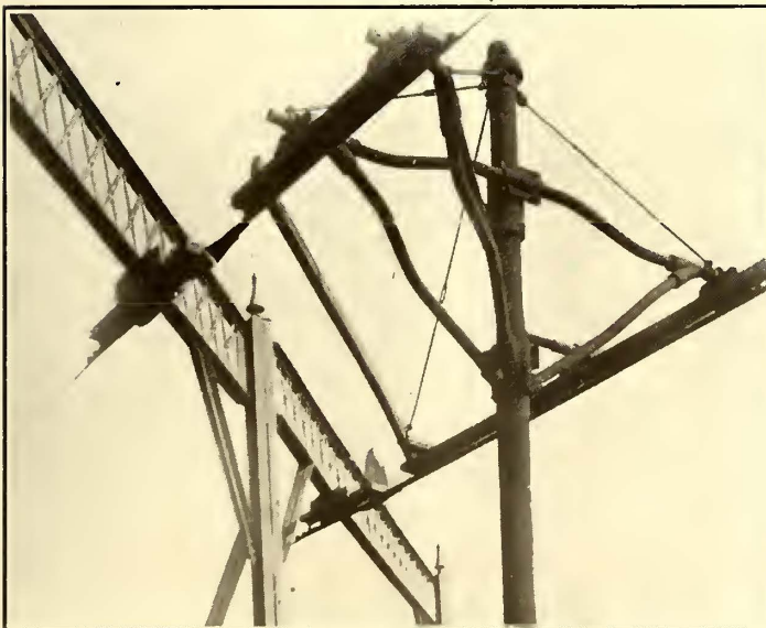
Brooklyn Line Department—Overhead Work at the Washington Avenue Bridge
