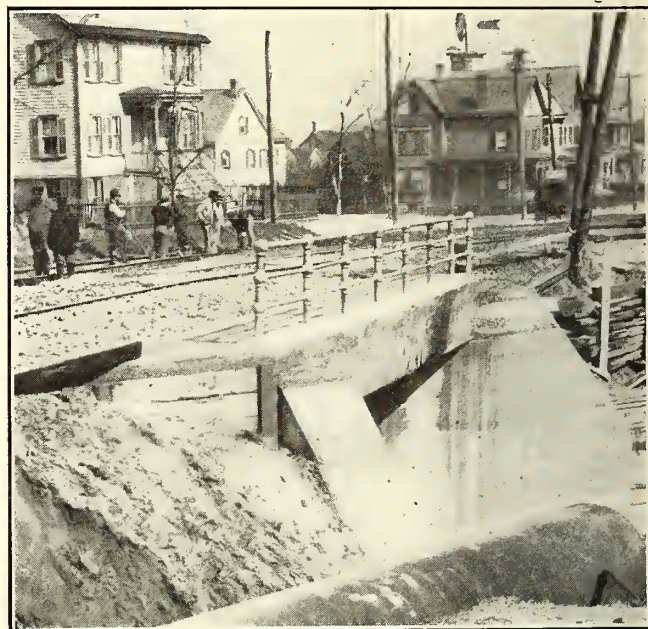
Fig. 14—Track Maintenance—Concrete Bridge Built in Freezing Weather
