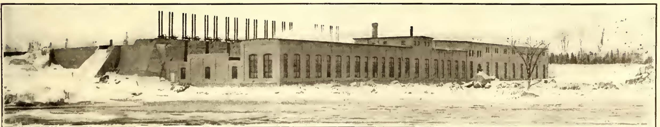
Winnipeg System—Downstream View of Hydroelectric Station
