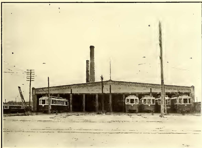
Winnipeg System—Repair Shops
