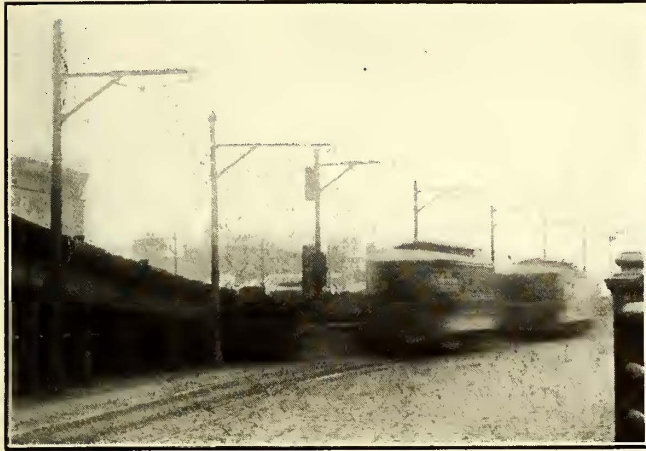
Brooklyn Line Department—Double Trolley Wire on Brooklyn Bridge Incline
