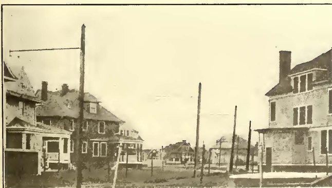
Brooklyn Line Department—Overhead Work on Right-of-Way in Suburban Territory
