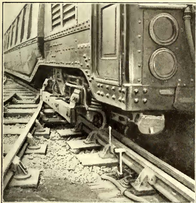
London Underground—Showing Position of Train Stop Outside the Rails
