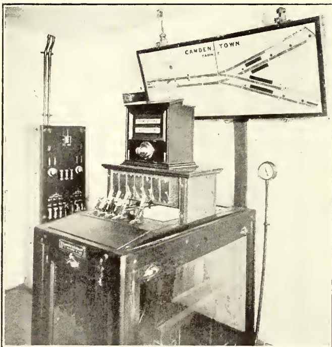
London Underground—Signal Interlocker and Illuminated Diagram at Camden Town
