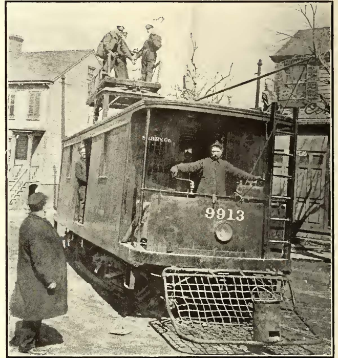
Brooklyn Line Department—Running Trolley Wire from a Car in a Suburban Town
