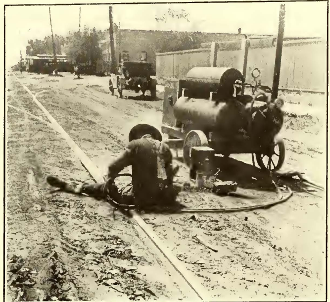
Bonding with Oxy-Acetylene Torch
