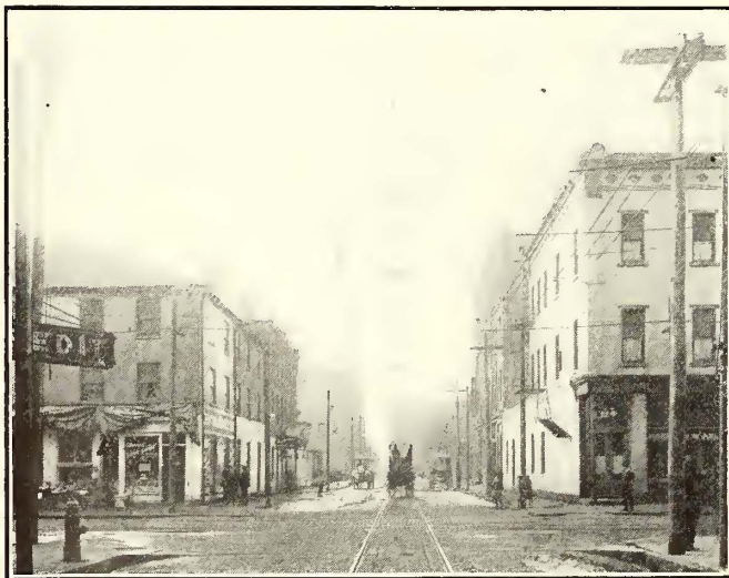
Southern Cambria Railway—Overhead Construction on City Streets
