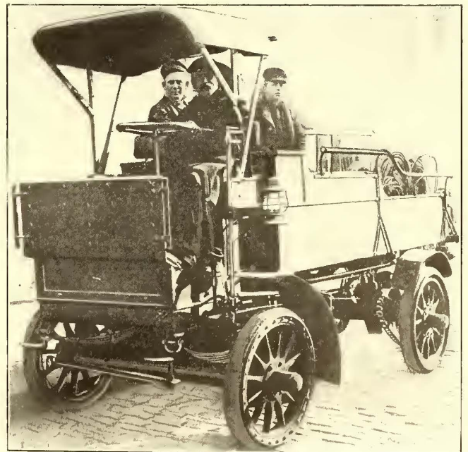
Brooklyn Line Department—Automobile for the Lighting Repair Gang
