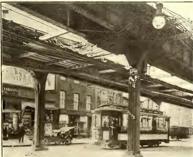
Brooklyn Line Department—Iron Bar and Feeder Construction on Flatbush Avenue
