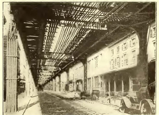
Brooklyn Line Department—Feeders Led up Pillars on Both Sides of the Street at Hudson Avenue Station
