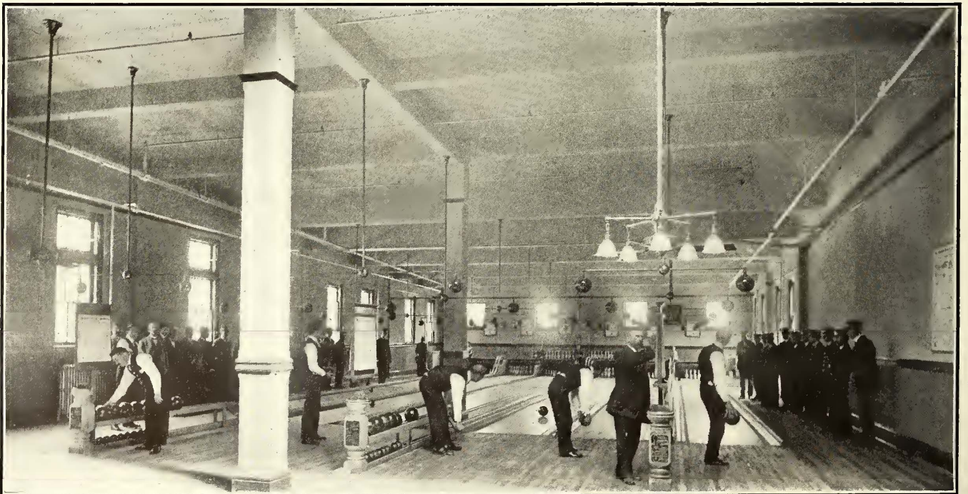
Park Terminal Car House—The Bowling Alley, Showing Also the Concrete Beam Construction on the Second Floor and Lighting Scheme
