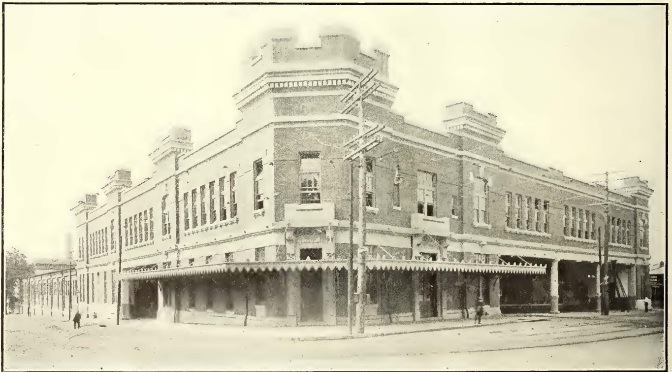
Park Terminal Car House—General View, Showing the Parapet Style of Construction
