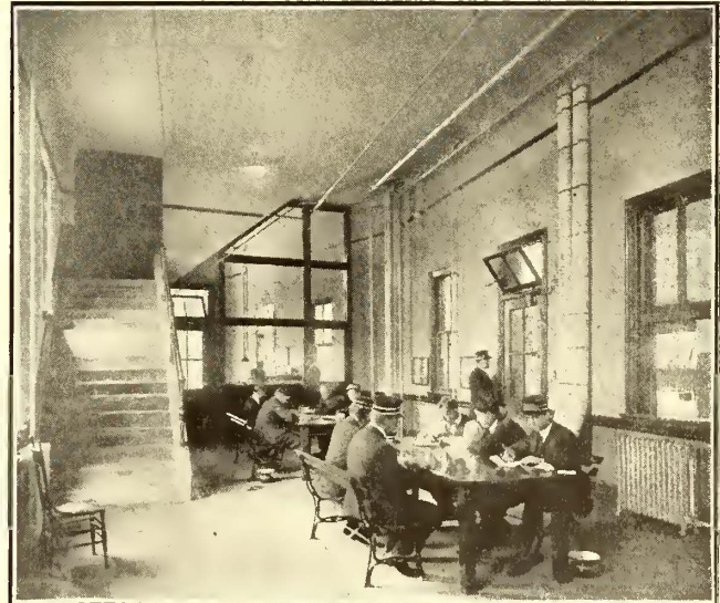
Park Terminal Car House—Concrete Stairway from Crew Room to Upper Floor
