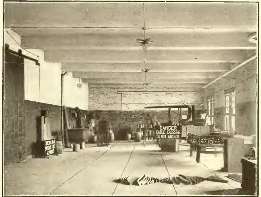
Brooklyn Line Department—A Portion of the Paint Shop, Showing the Lighting with Vapor-Proof Five-Lamp Clusters
