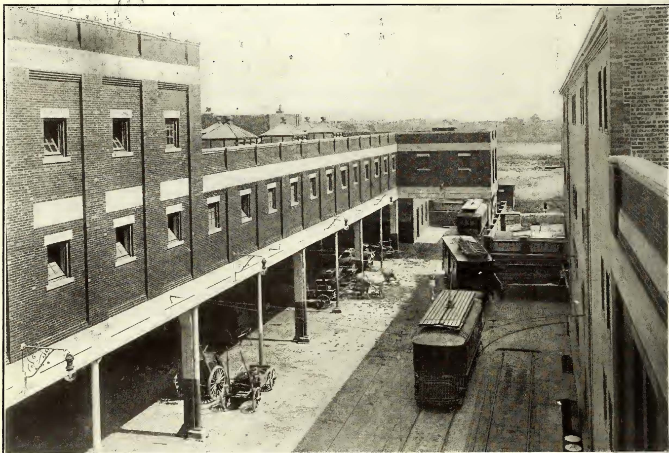
Brooklyn Line Department—A View of the Open Passageway Between the First and Second Buildings, Showing the Wagon Shelter Under the Stable on the Left and the Delivery Tracks and Scale on the Right
