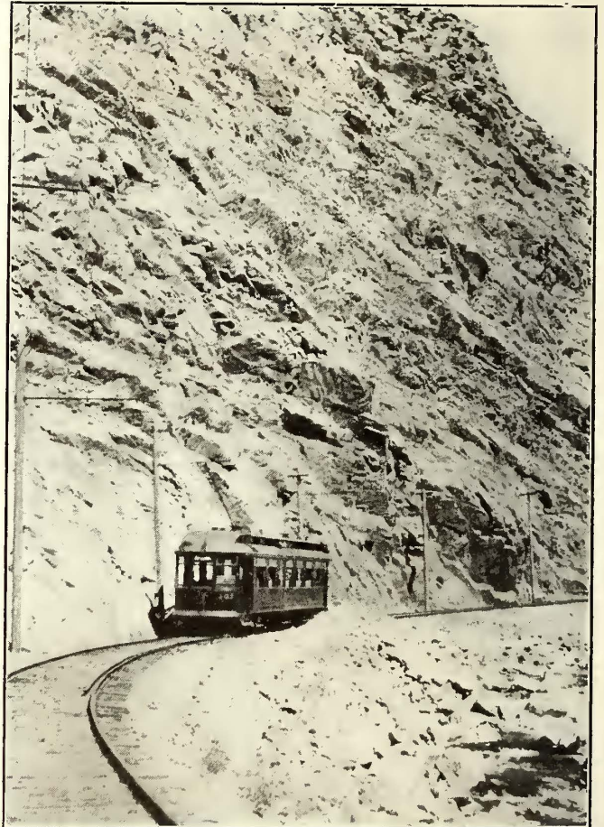
Ogden Rapid Transit—Ogden Canyon Line
