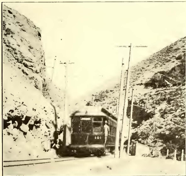
Ogden Rapid Transit—Ogden Canyon, Showing Construction Adjoining County Road
