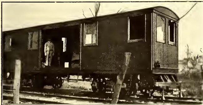
Reading Power Improvements—Portable Substation
