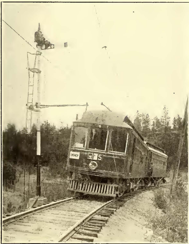
Fig. 7—Washington Water Power Company Signals—Home Signal and Automatic Stop Arm in Stop Position
