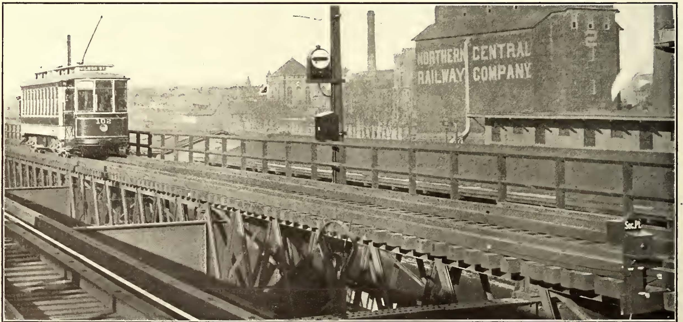
Signals in Baltimore—Stop Indication and Section Point
