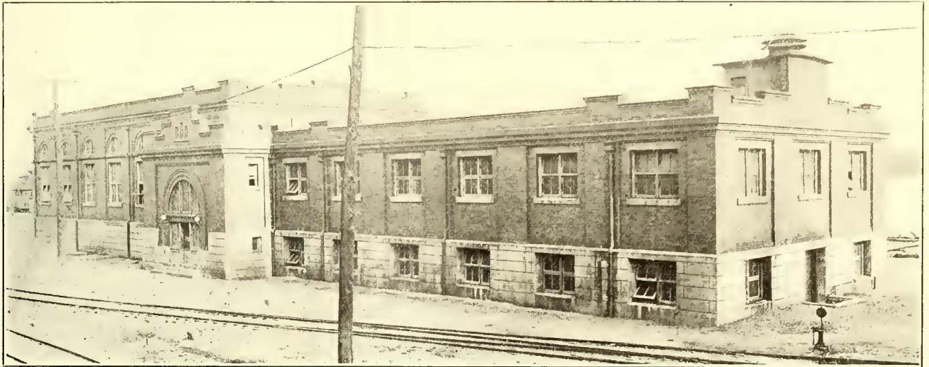
Fig. 3—Detroit Tunnel—View of the Converter Station
