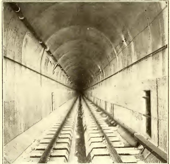
Fig. 5—Detroit Tunnel—Track Construction in the Tunnel
