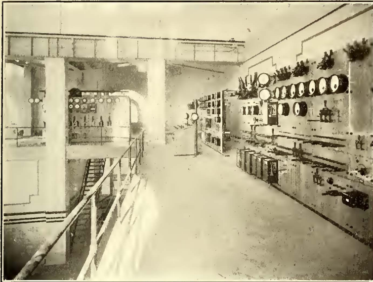
Southern Pacific Power Station—Switchboard from South End of Gallery
