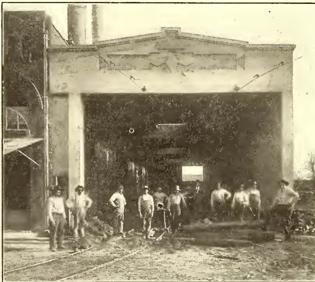
New Concrete Car House in Corsicana
