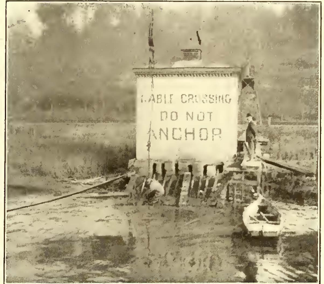
Fig. 6—Harlem Cables—Diver Cutting Servage Straps
