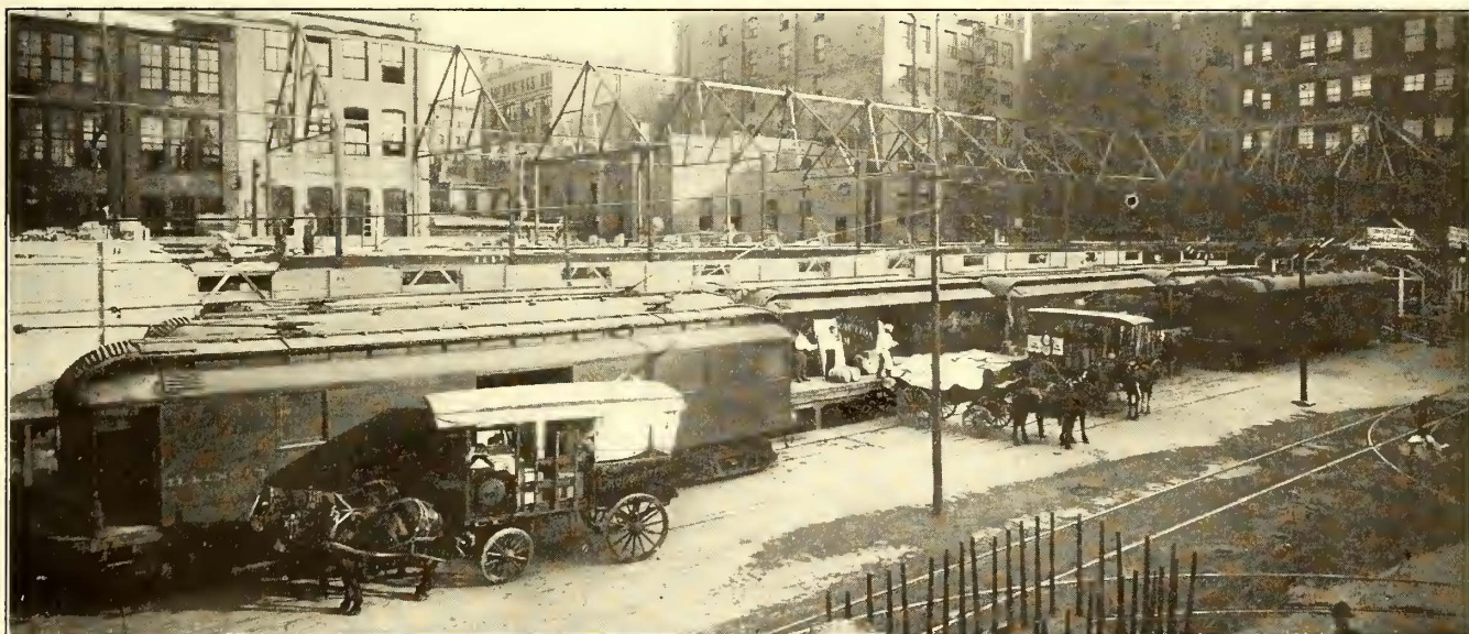
Freight and Express Terminal Under Construction in St. Louis
