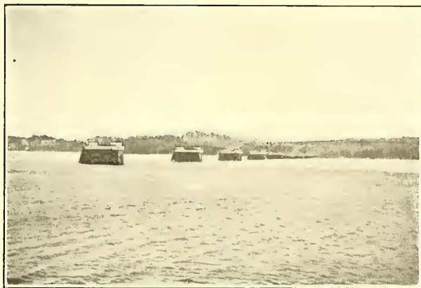
Connecticut River at Point Where Cable was Laid.
