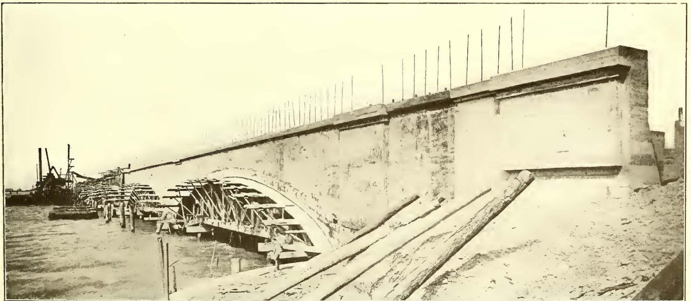
Galveston-Houston Railway—Concrete Causeway, View Taken During Construction
