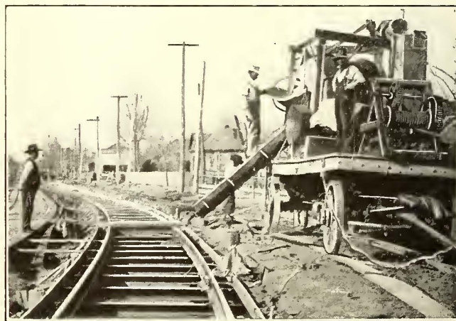
Fig. 4—Oklahoma Track—Concreting Steel Tie Track Direct from Mixer
