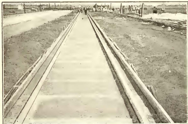
Fig. 3—Oklahoma Track—Steel Tie Construction Ready for Paving
