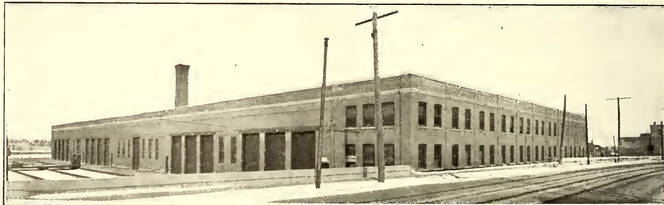
Fig. 1—Syracuse Shops—General View Looking Along Southern Transfer Table and the Wolf Street Side
