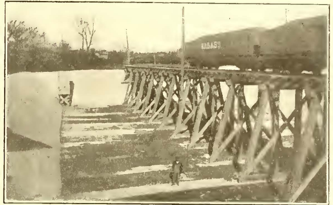
Coal Storage Pit and Trestle
