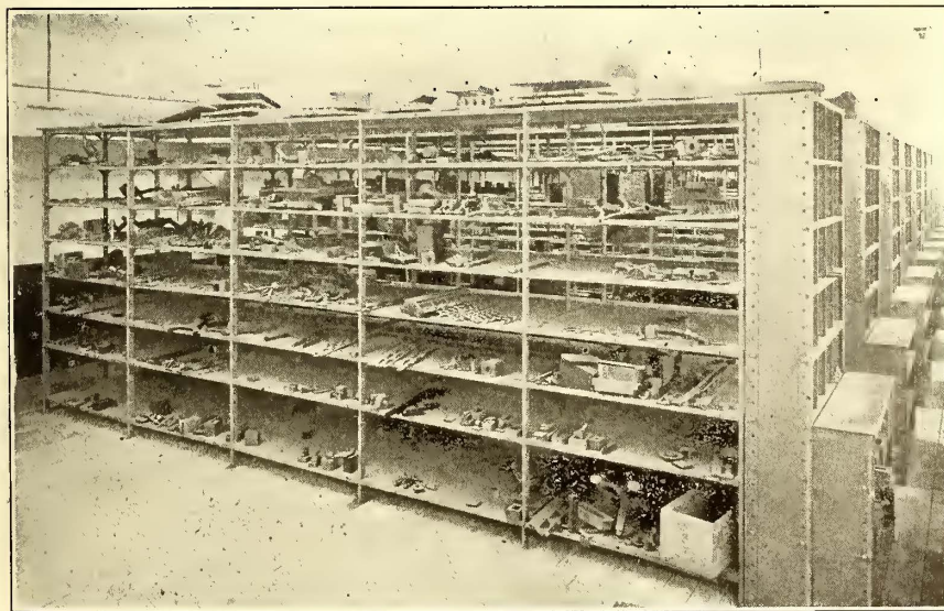
Chicago Railways Shops—Pattern Storage Room with Steel Adjustable Shelving
