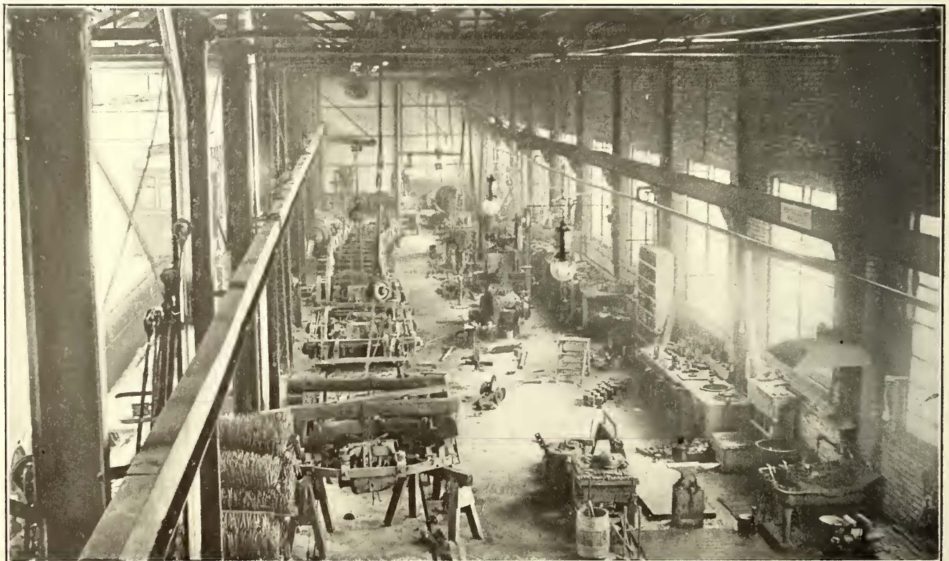
South Bend Shops—Machine Shop Section
