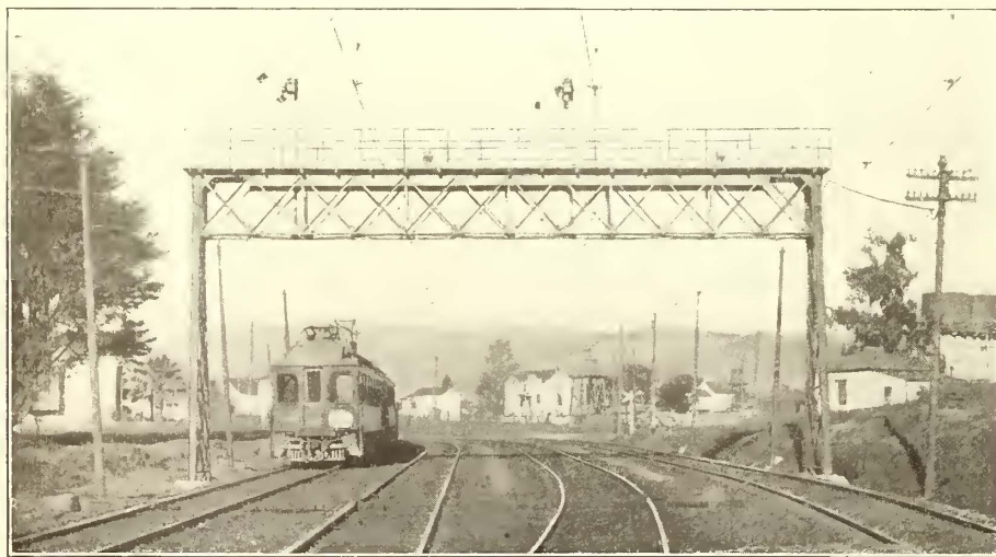
Key Route Signals—Signal Bridge at Tower No. 3
