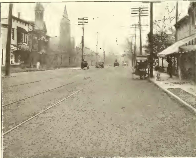
Brick Paved Street with Pitch Filler
