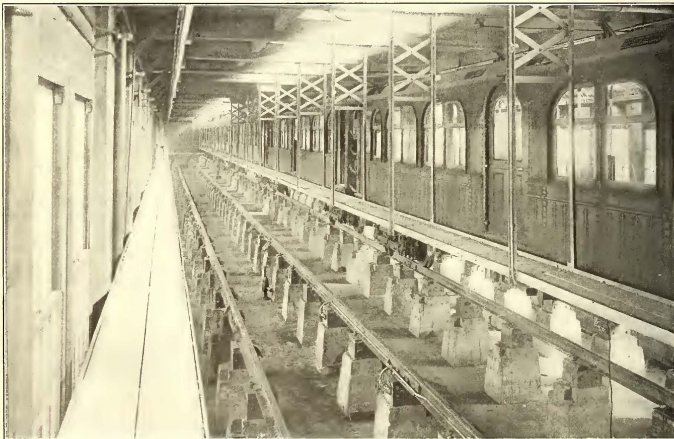
Hudson & Manhattan Railroad—View of Inspection Shed, Showing Suspended Walkways
