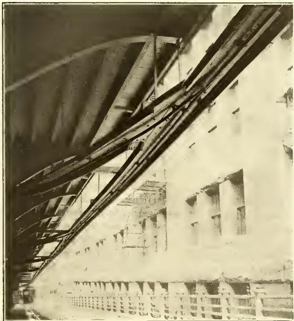
Double-Bar and Single-Bar Overhead Construction at the Brooklyn Bridge Terminal
