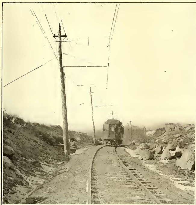
Fig. 15—Shore Line Railway—Pull-Off Construction on Curve Between Guilford and Saybrook
