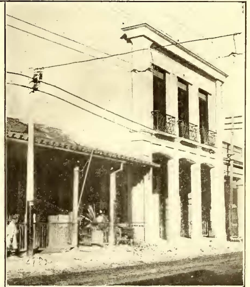
Dwelling House and Substation
