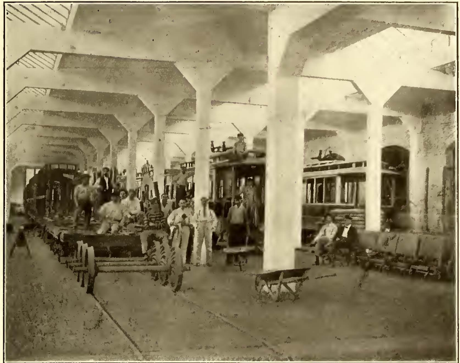
Havana Electric Railway—Truck Shop
