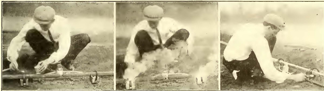
Figs. 1, 2 and 3—Process of Thermo-Welding Rail Bonds
