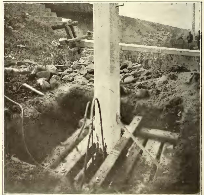
Pennsylvania Railroad—Setting Reinforced Concrete Pole and Grillage with Air Jet
