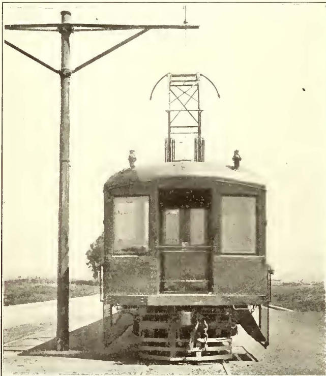
Southern Pacific Electrification—End View of Steel Motor Car, Showing Roller Pantograph
