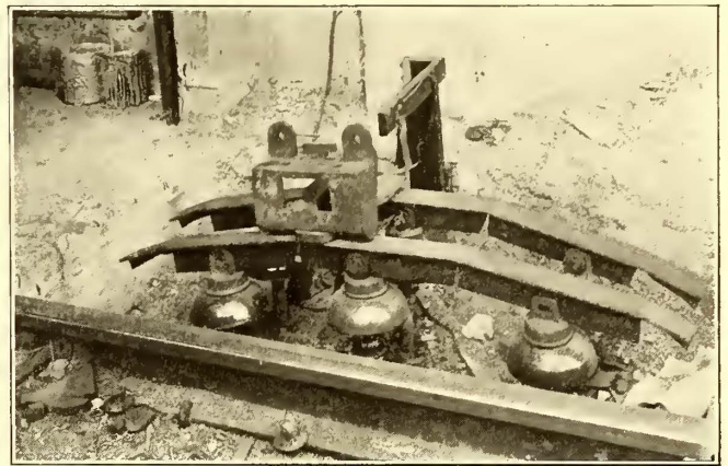
Hudson Shops—Third-Rail Shoe Tell-tale Outside of the Inspection Shop
