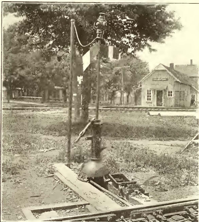
Illinois Traction Signals—Switch Circuit Controller and Lighting Connection for Switch Lamp
