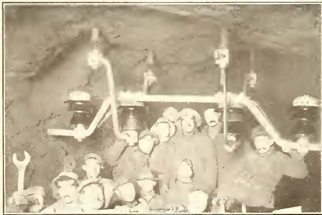
Hoosac Tunnel—Erecting Tunnel Catenary Brackets
