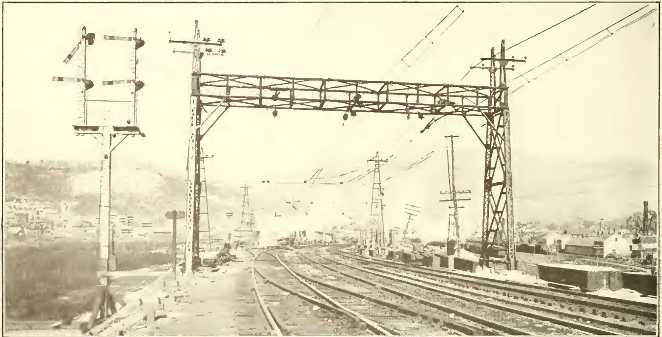
Hoosac Tunnel—Anchor Bridge at East End of North Adams Yard
