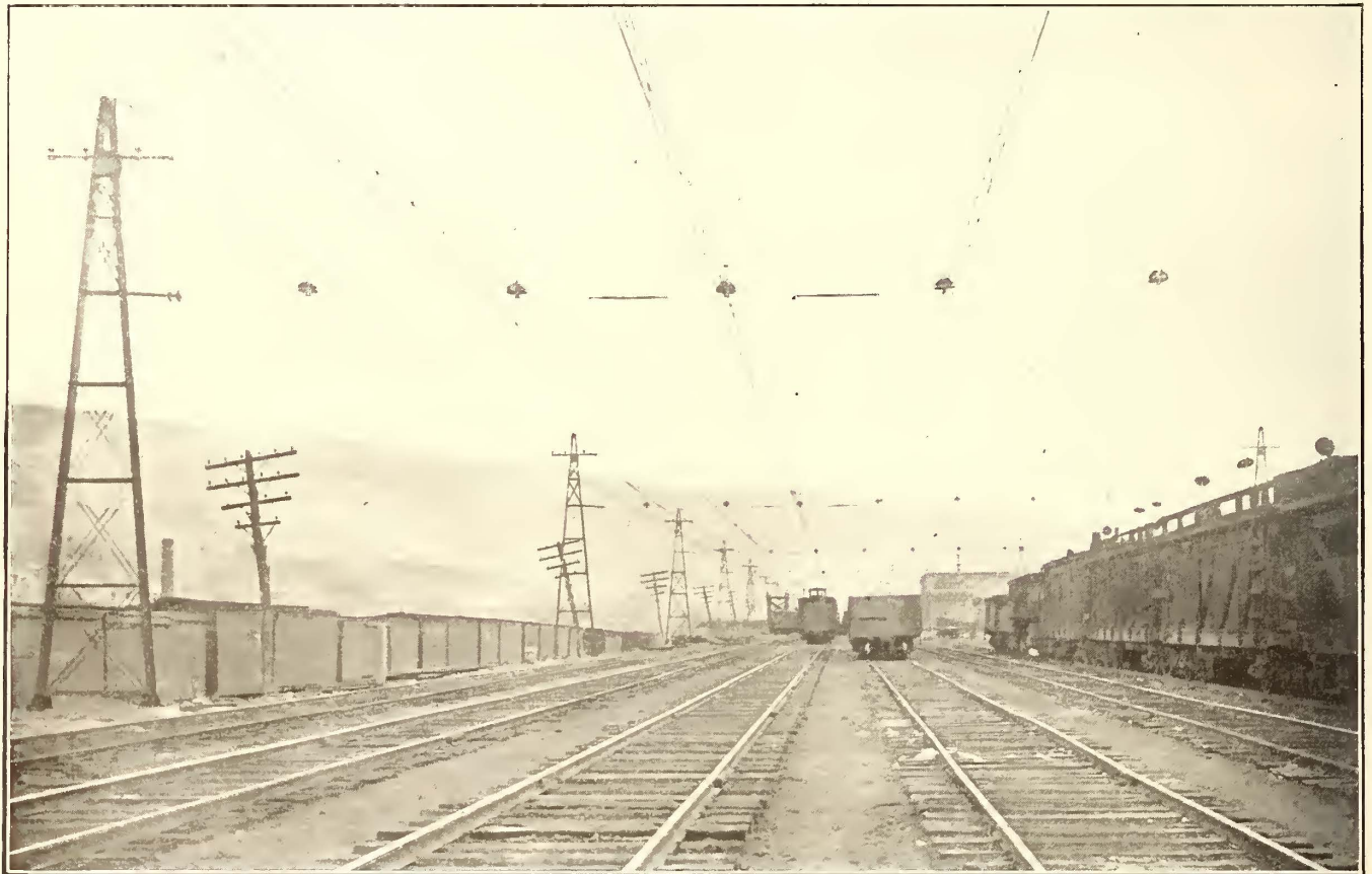
Hoosac Tunnel—Cross-Catenary Construction in North Adams Yard
