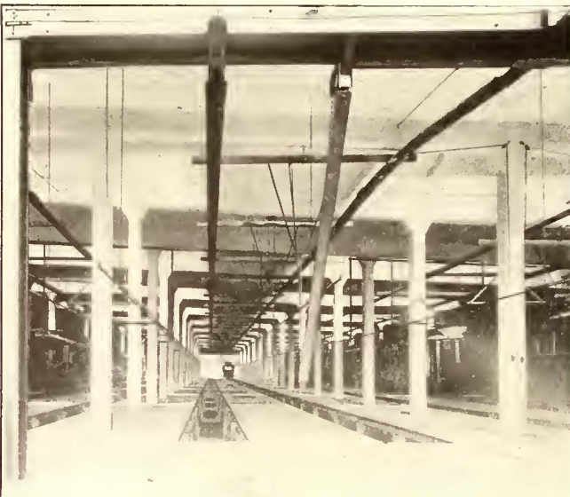
Bridgeport Carhouse—View Through a Storage Bay
