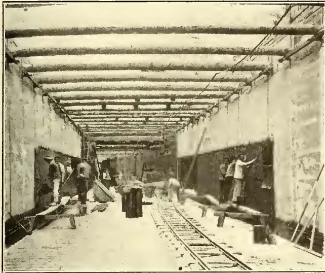
Schöneberg Subway—Waterproofing the Outer Concrete Walls
