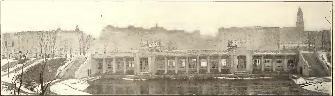
Schöneberg Subway—Side View of Open Cut Station Through the Stadtpark, Showing the Artistic Treatment of the Structure, Stairways for Crossing Over the Railway, Statuary, etc.—The Subway Portal Is at the Extreme Left
