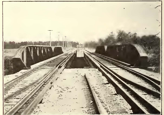
Aurora, Elgin & Chicago—Example of a Standard Through Girder Bridge
