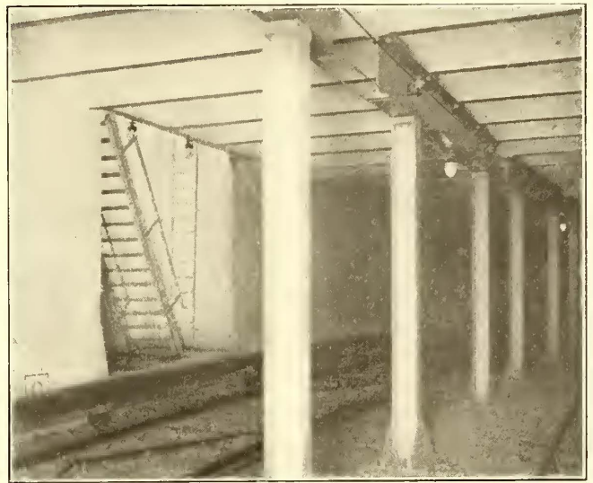
Schöneberg Subway—Emergency Exit and Ventilating Shaft Combined
