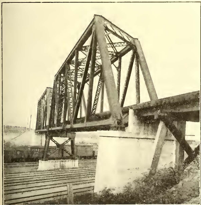
Aurora, Elgin & Chicago—Bridge Over Steam Railroad Tracks at West Chicago
