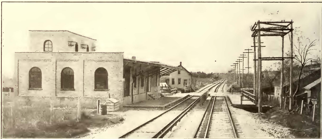
Aurora, Elgin & Chicago—Combination Depot and Substation
