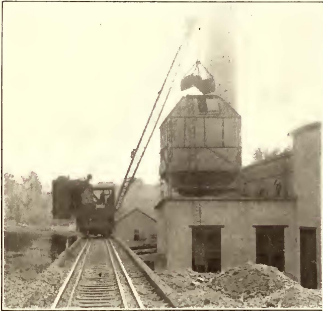
Worcester Power—Coal-Handling Machinery
