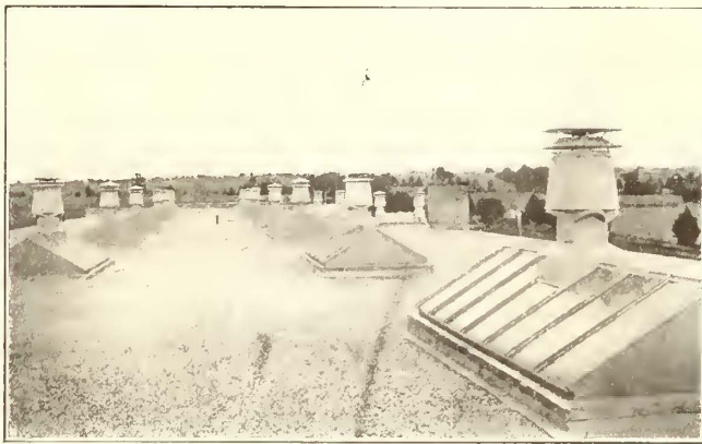
Rockford Shops—Skylights and Ventilators in Roof
