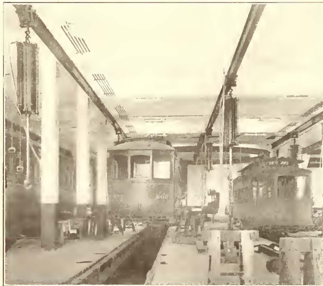
Rockford Shops—General Repair Shop
