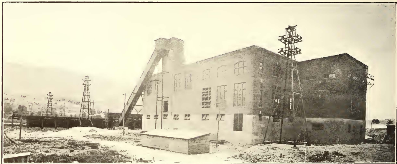
Hoosac Tunnel Power Station—Exterior View Showing Coal Conveyor and Outgoing Transmission Line
