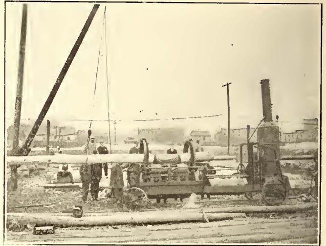
Pole-Preserving Machine in Service
