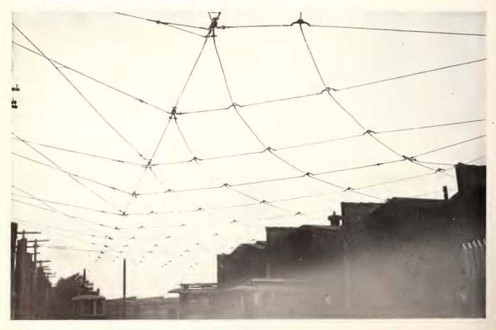
Another Example of Well-Aligned Overhead Construction as Installed in Front of the Plank Road Storage Carhouse,
