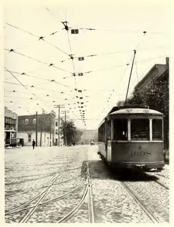
Overhead Construction with Numbered Switches in Front of West Hoboken Carhouse
