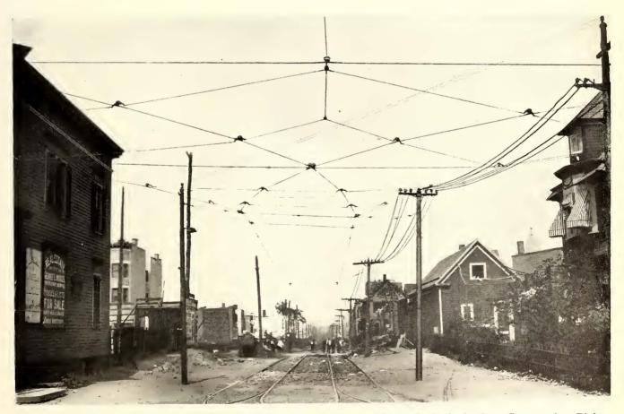
Fixed-Angle Overhead Construction in Place at Fourth Street, Union Hill, at the End of a Span-Construction, Right-of-Way Line
