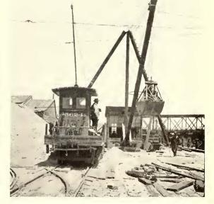
Views of Stationary Derrick Delivering Ballast to Work Car at Passaic Wharf
