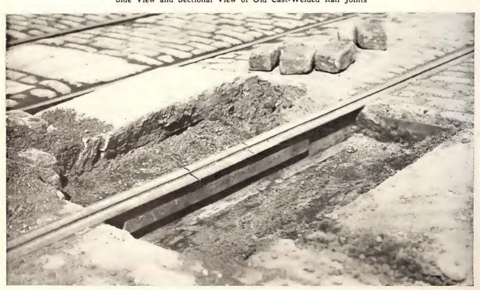
View of Old Cast-Welded Rail as Rehabilitated by Means of Insert Piece and Electrically-Welded Joint
