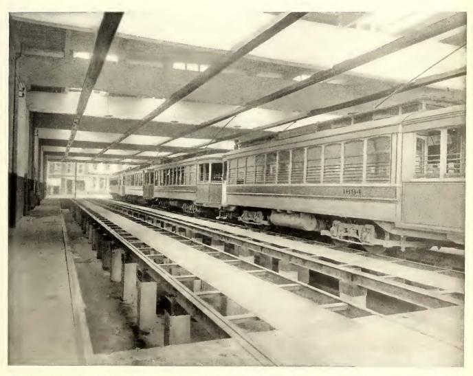
Interior of the West Hoboken Carhouse, Showing the Style of Open Pits with Metal Devil Strips, Roof Construction and Lighting, Etc.
