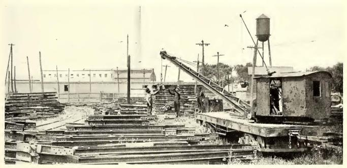
Handling Special Work with Old-Type Crane Car
