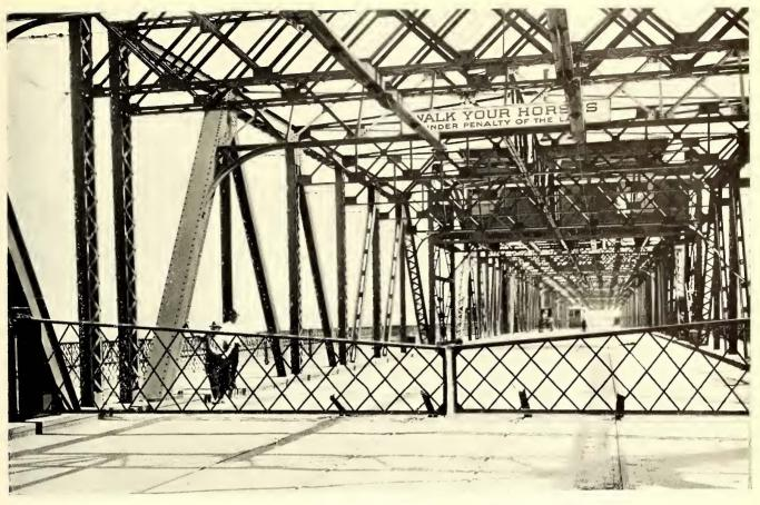
Lift Rails at Draw of Plank Road Bridge Over the Hackensack River
