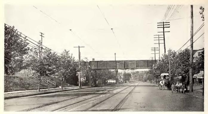
An Example of Paving in Newark, Where the Railway Company Was Permitted to Use Granite Along the Rails, the Rest of the Street Being Paved with Asphalt
