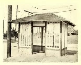
Shelter Station at Morsemere—The Sides Are Constructed Principally of Glass
