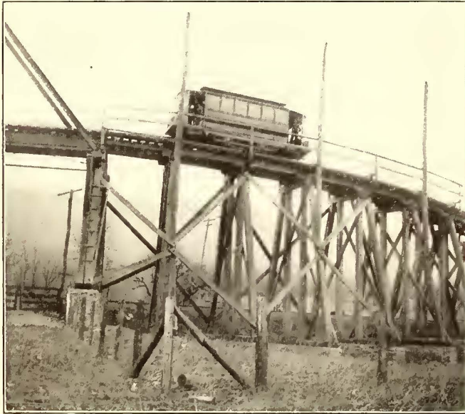
Type B Car of 60-hp Mounting a 10 per Cent Grade on Schuylkill & Dauphin Railway
