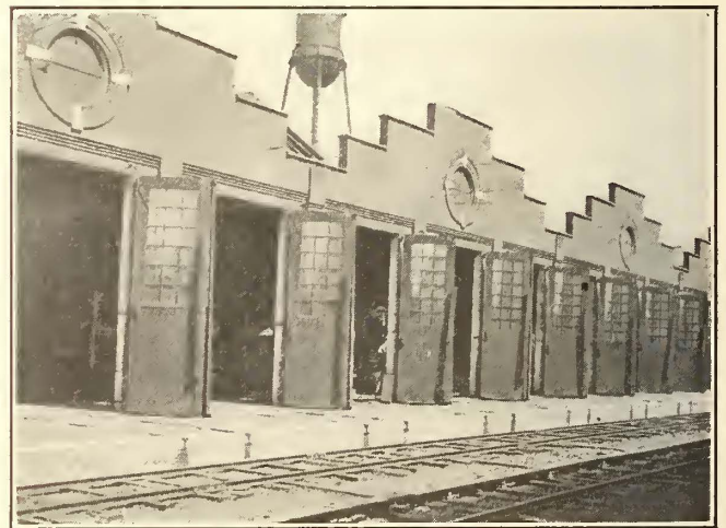
Fig. 6—Buildings and Structures—Wooden Swinging Doors for Carhouse
