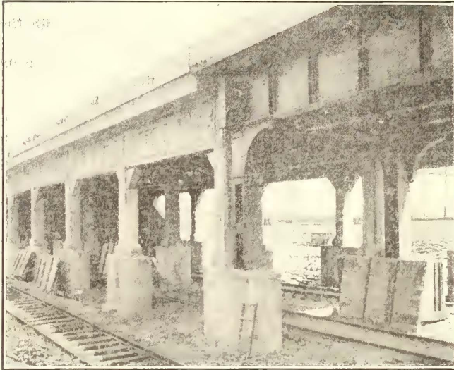
Fig. 1—Buildings and Structures—Steel Viaduct Inclosed in Concrete
