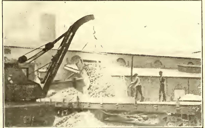
Key Route Power Plant—Dumping Excavated Earth on Flat Car
