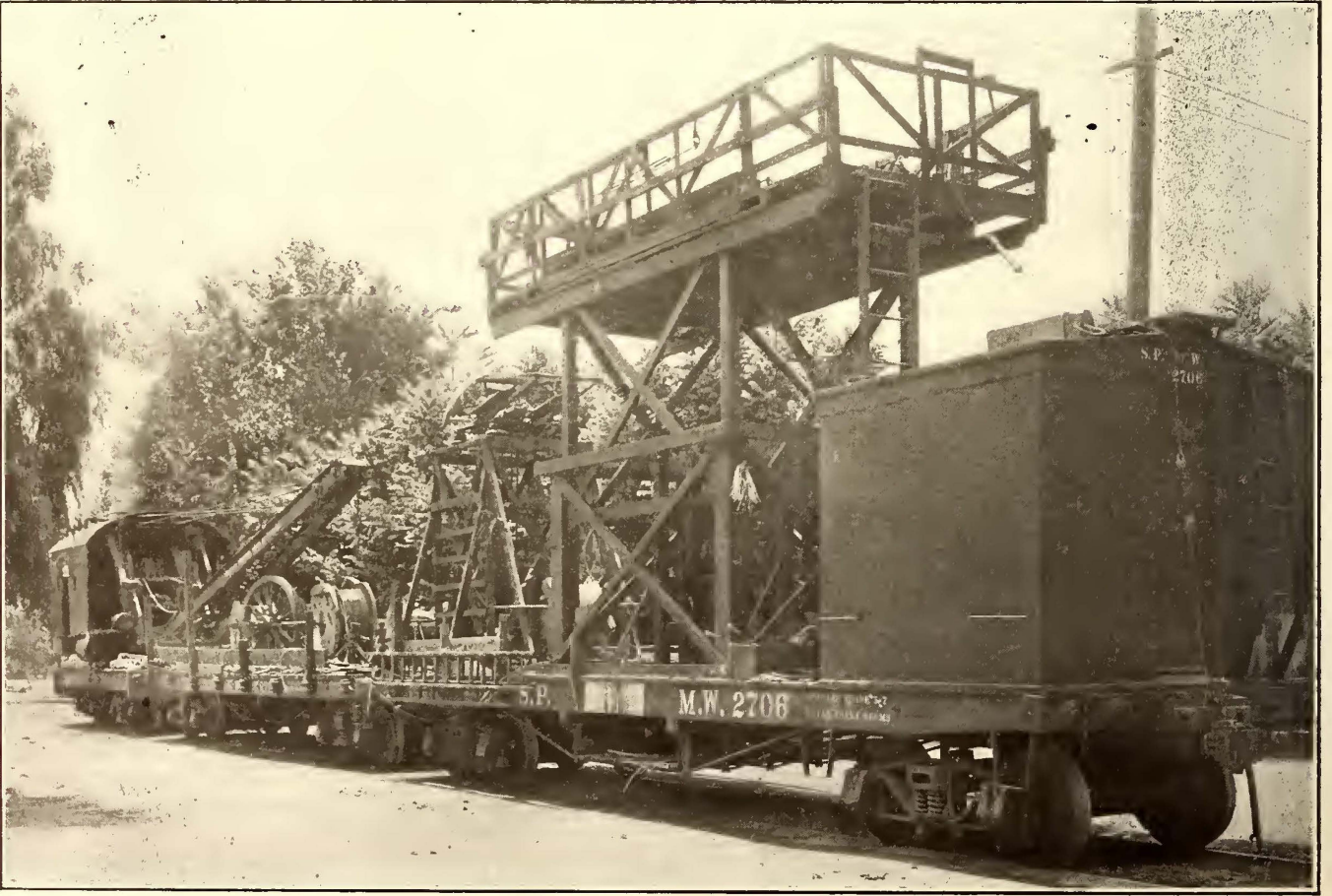
Fig. 34—Southern Pacific 1200-Volt Lines—Standard Construction Train Installing Overhead Work
