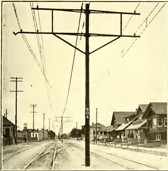
Fig. 25—Southern Pacific 1200-Volt Lines—Overhead Construction at Cross-Overs
