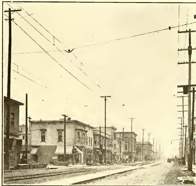
Fig. 21—Southern Pacific 1200-Volt Lines—Cross-Span Construction on Tangents
