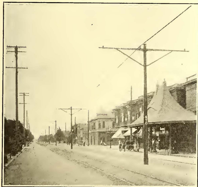
Fig. 19—Southern Pacific 1200-Volt Lines—Center Pole Construction on Tangent Track in City Streets
