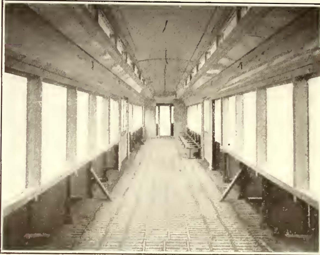
Interior View of Philadelphia Elevated Car, Showing Completed Ceiling, Part of Seat Framing, Etc.
